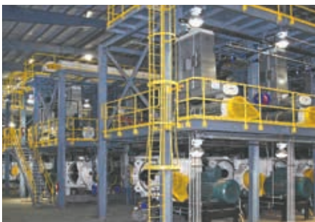
Installation of ANDRITZ Pellet mill PM30
